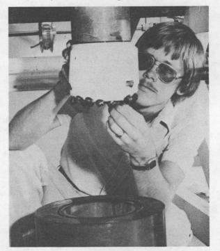
DURING THE HEIGHT of Sandia's drilling R&D activities, Dave Glowka (6252) often was found examining drag bits before testing in the Bit Hydraulics Facility. During testing, the rotating bit was situated inside a transparent plastic hole that simulated a borehole.
